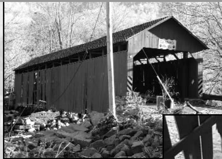
Sonestown Covered Bridge and closeup of flood damaged siding.
