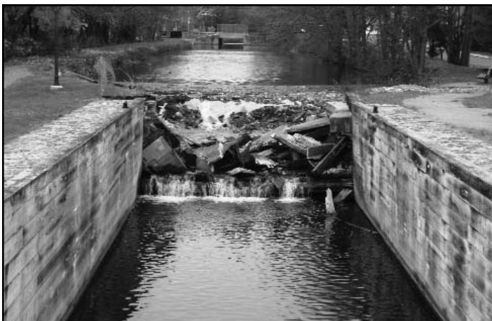
Fall gate at Lock #23 of the Lehigh Canal at Walnutport before (above) and after (below) it sustained significant damage as a result of a tropical storm in late August 2011.
