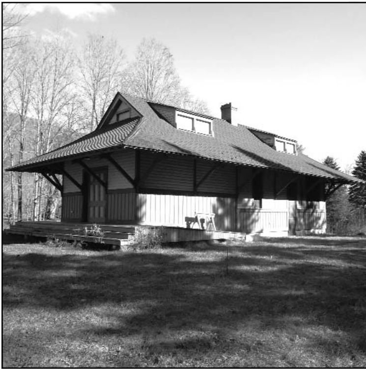
Photo courtesy of Erin Hammerstedt, Preservation Pennsylvania.
