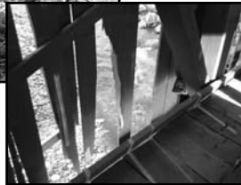
Sonestown Covered Bridge and closeup of flood damaged siding.
